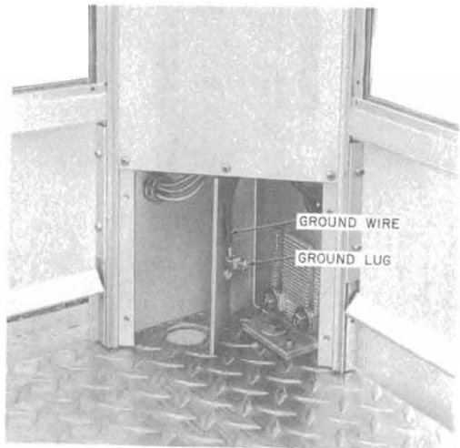
Fig. 6—Grounding Screw in KS-19580 Booth
